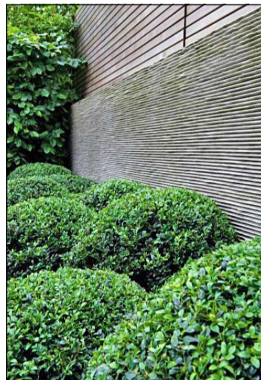
Textural wall: porcelain tiles, built up in layers, create a pleated effect
