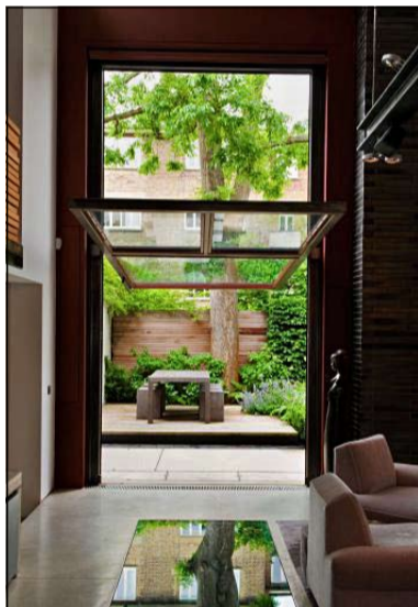
Glass canopy: a cantilevered window provides shelter at the entrance
